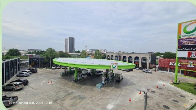
Bangchak Service Station Chaengwattana
