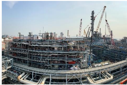
PTU – Equipment, Piping & Structure Installation
