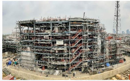
SAF – Equipment, Piping & Structure Installation
