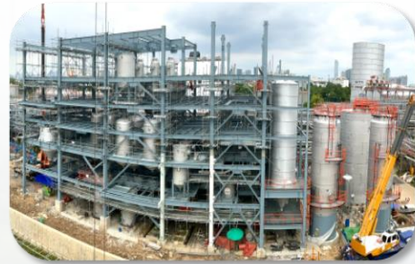
PTU – Equipment, Piping & Structure Installation
