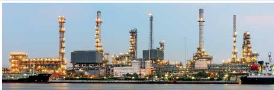
Refinery Business (with a refining capacity of 120,000 barrels per day)
