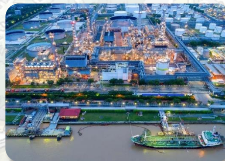
Phra Khanong Refinery
