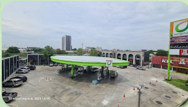
Bangchak Service Station Chaengwattana
