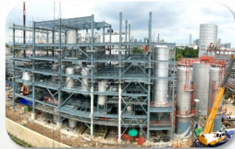
PTU – Equipment, Piping & Structure Installation
