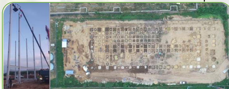
Construction Progress 40% (as of JUL24)
